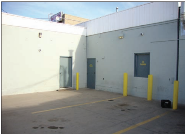
In this case the designer has eliminated roof access and installed secure doors and CCTV on the walls to protect the property.
