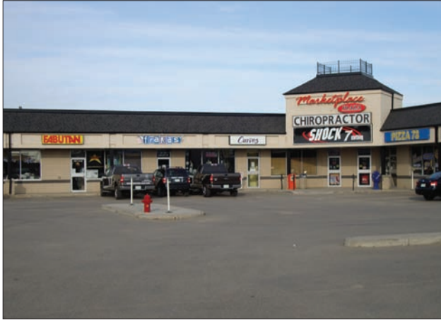
This commercial mall is cleaned and walls are graffiti-vandalism-free.
