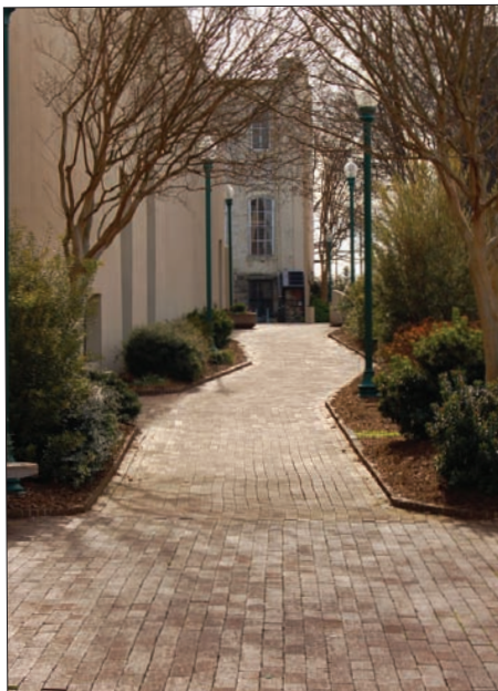
High, pole-mounted lighting on both sides of this pedestrian walkway ensures even distribution of illumination along the entire path.
