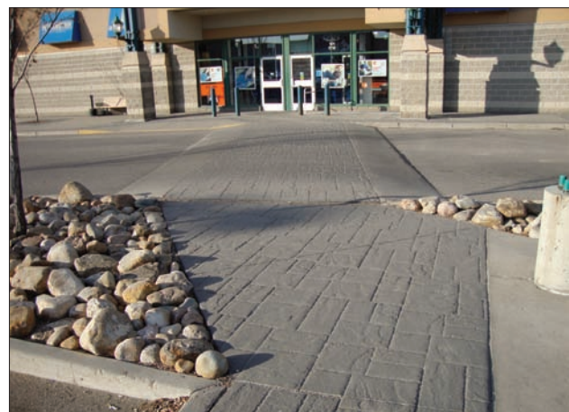
The designer has changed the grade on a walkway to illustrate a transition from a parking lot, over a roadway, to a storefront.
