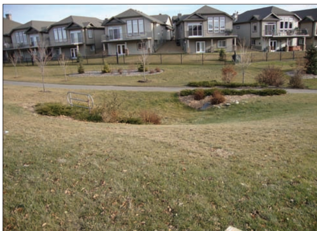
Natural surveillance is maximized here through landscaping islands, see-through wrought-iron-type fencing, and low foliage.
